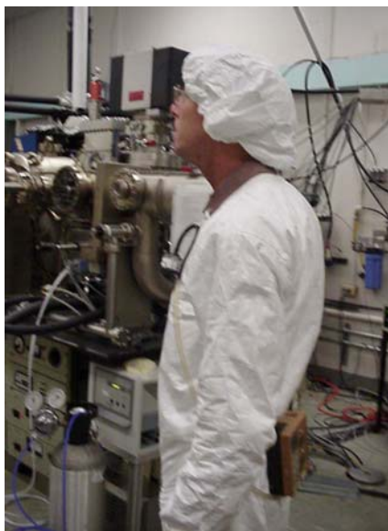
Photo 3. Engineer wearing an air sampling pump and filter cassette before performing maintenance work on the MBE
